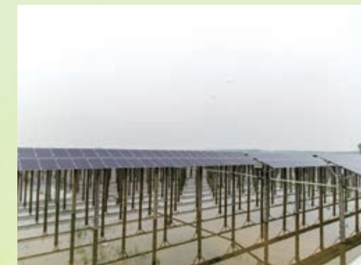
Shouxian Solar Farm 壽縣光伏電站
